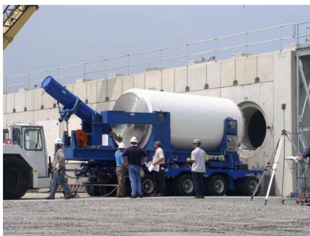
NUHOMS ® used fuel dry storage system at the site of a US utility
