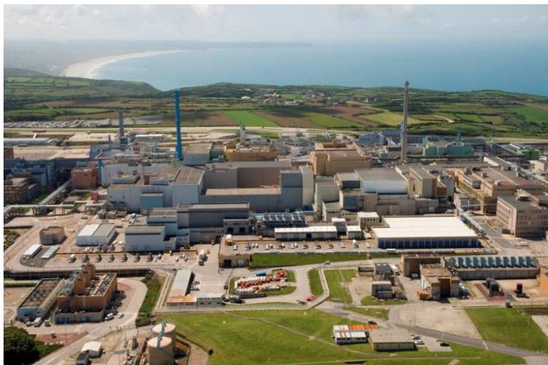
Orano La Hague reprocessing plant in France
